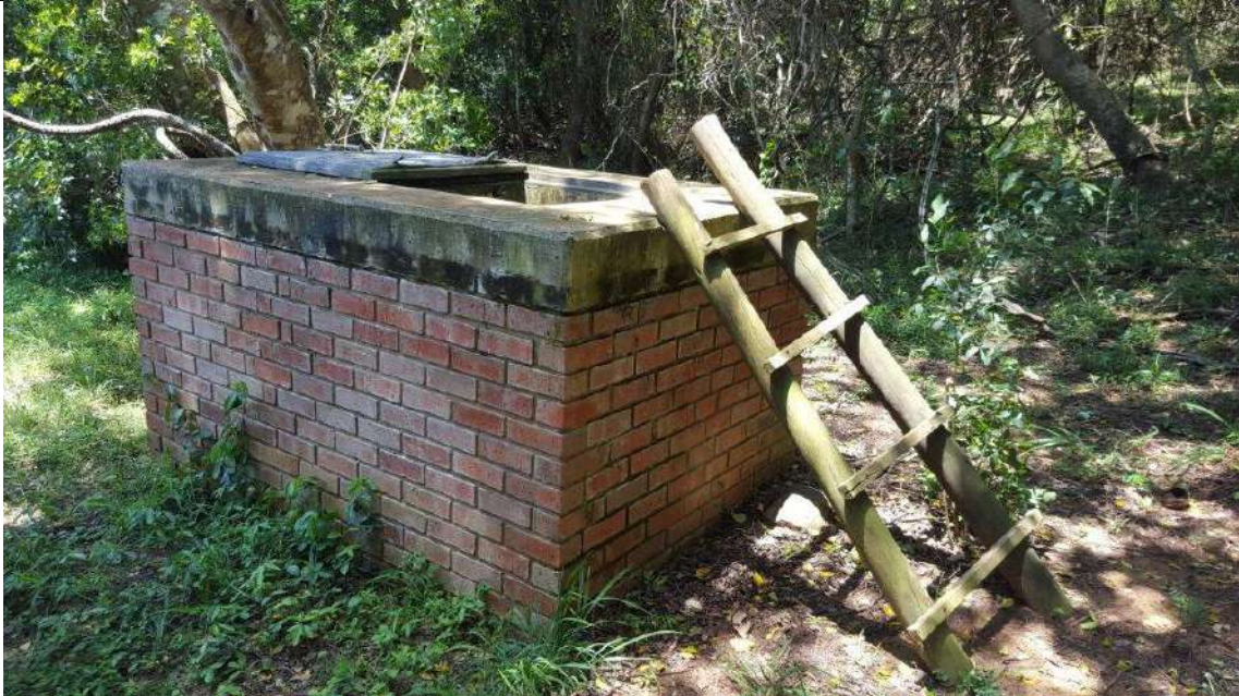
Borehole chamber at Bhangazi site
