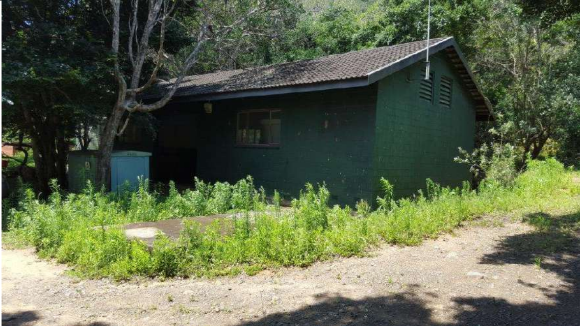
Water pumphouse at Bhangazi site
