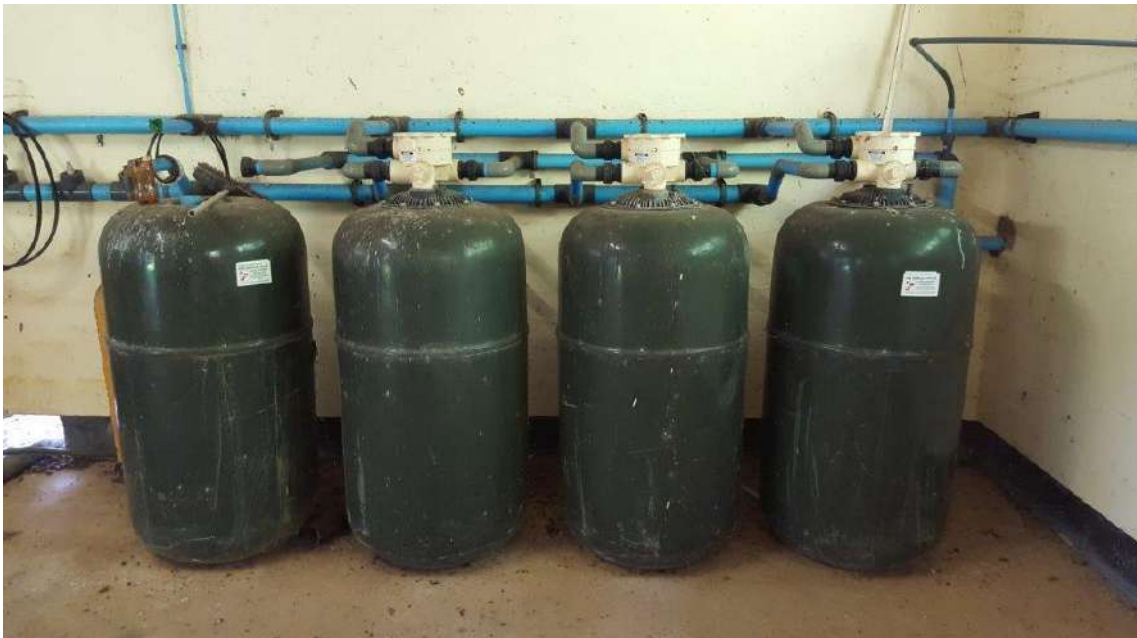
Old filters not in use at Bhangazi water pumphouse
