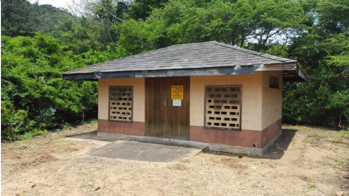
Existing substation at Bhangazi site with a reported capacity of 1,1MVA
