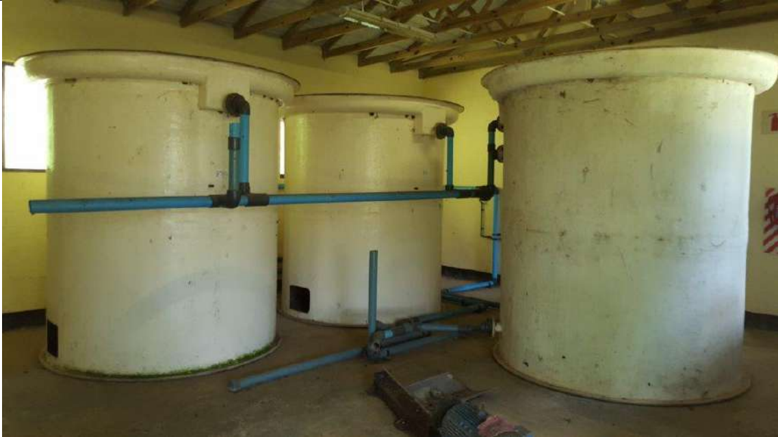
Old settling tanks not in use at Bhangazi water pumphouse
