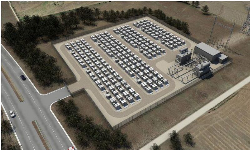
FIGURE 8-6 SOLARCITY'S TESLA BATTERY STORAGE FACILITY, HAWAII
